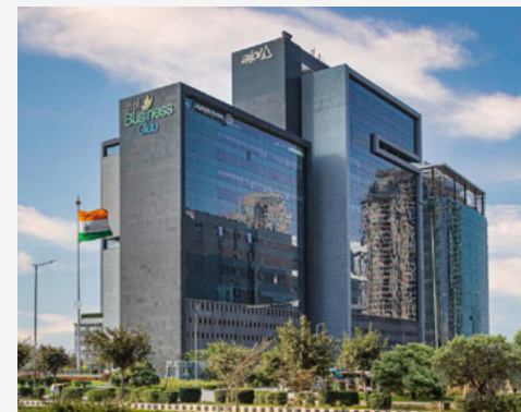
Milliman's occupancy of a GRIHA 4 Star and LEED Gold certified building contributes to sustainability efforts in India.
